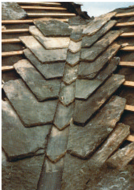
Figure 12 The heavy, flat sandstone flags of the South Pennines are suitable for lower pitches, and the detailing of the roof is simpler to accommodate their large dimensions. The chevron valley is an example of the craftsman's skill in forming a weather-tight roof.
