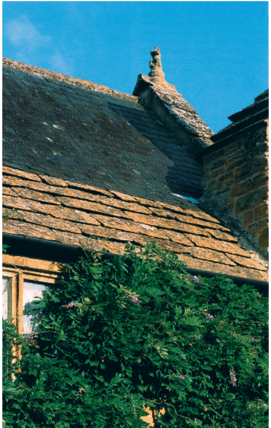
Figure 13 Eaves slating is a traditional roofing practice in some parts of the country. In some areas stone slate has been gradually replaced by other roofing materials such as metamorphic slate, and the stone slates at the eaves are a remnant of an earlier roofing material. The example shown here is in the village of Montacute, where the local Ham Hill stone slates have become increasingly scarce.
