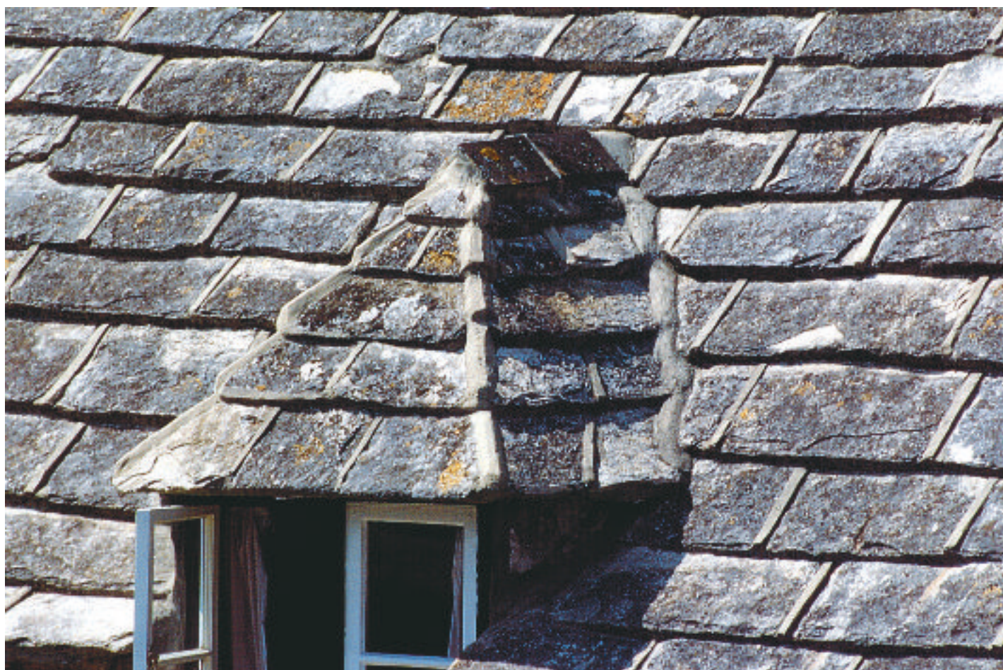
Figure 17 The misinterpretation of historic details and their modification with modern materials can cause difficulties. The cement pointing to this Purbeck stone slate roof is unsightly and technically problematic.
