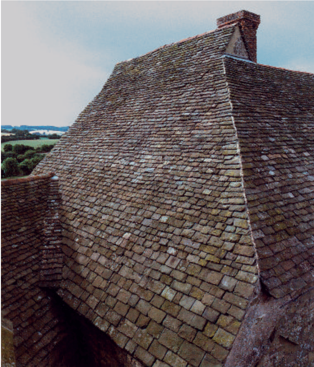
Figure 18 The hip of the roof at Stokesay Castle, Shropshire has been formed with lime mortar, which disguises the introduction of a lead soaker beneath to ensure that the roof is weather-tight.
