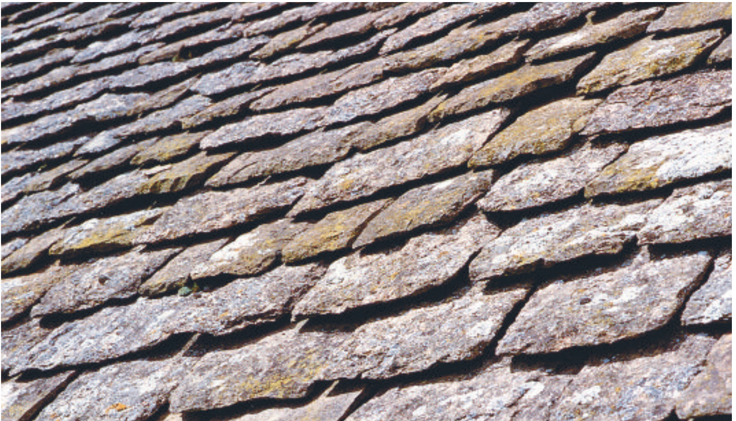
Figure 16 Langley Chapel, Shropshire. This Harnage stone slate roof includes both sandstone and calcareous sandstone, which overlie each other in the same quarry. The calcareous sandstone is identifiable by the presence of white lichen.
