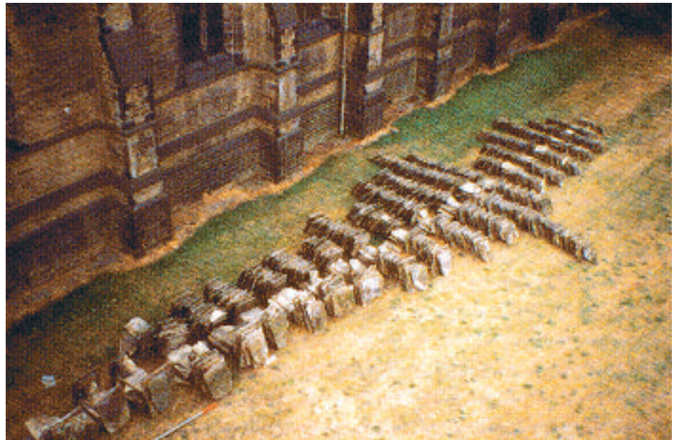
Figure 8 Stone slates removed from the roof and sorted according to size. The roofer will now be able to calculate the amount of new material required for reroofing.
