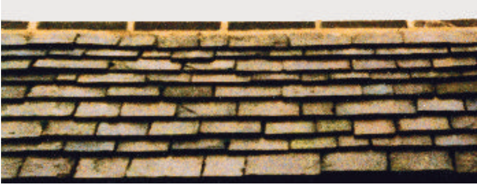
Figure 15 'Pigs' (where a long margin is visible above a short one) indicate a failure to maintain adequate head lap and are evidence of poor workmanship, as this roof in West Yorkshire shows.
