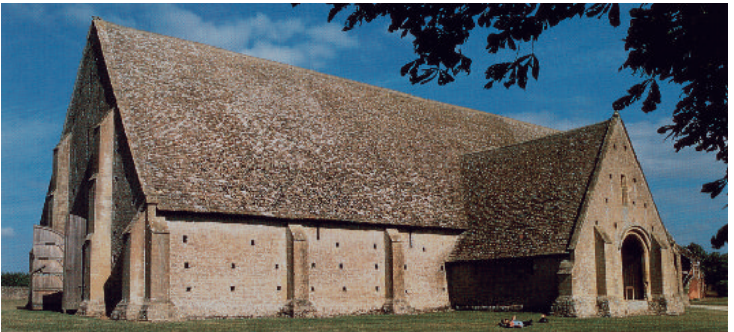
Figure 19 These small Cotswold stone slates have been laid at a steep pitch to form the huge roof of Great Coxwell Barn, Oxfordshire.
