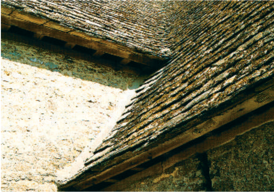
Figure 11 The limestone slates of the Cotswolds, which are lighter and smaller than most sandstone slates, require a steep pitch and can accommodate curves in swept valleys.
