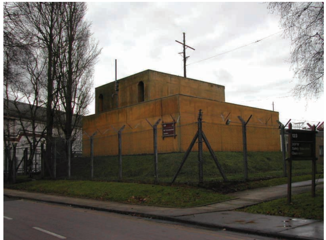
The Hardened Telephone Exchange
