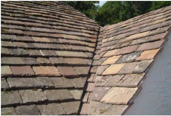
Fig. 49. In Wales and the Welsh Marches, stone valleys are traditionally constructed by laying a set of stone-slates underneath the slates in the adjacent slopes. These are known as Welsh valleys. Photo: John Goom.
