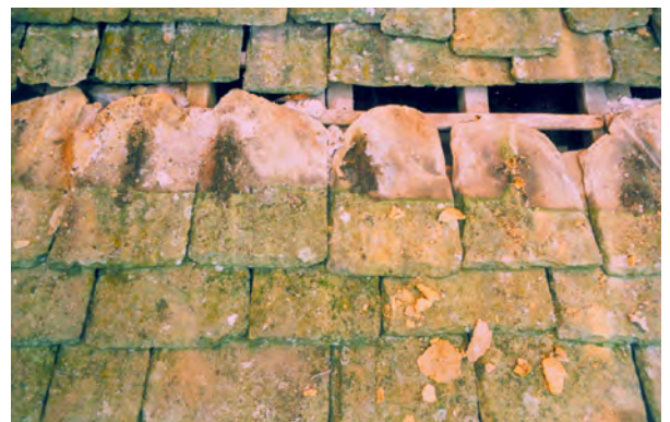
Fig. 19. Carboniferous, Pennant Sandstone roof of St Brievals Castle in the Forest of Dean. This formation in the Coal Measures Group has been worked for roofing here, around Bristol and the South Wales Coalfield. Photo: Terry Hughes
