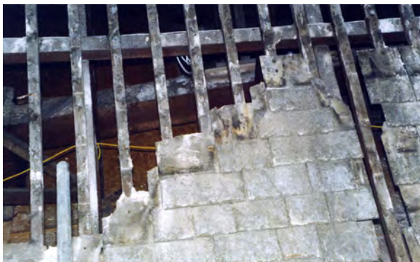
Fig. 36. In the South West rag slates are nailed directly to the rafters. The rafters are set closer together than in normal slating but even so some slates are too narrow to lie over two rafters. In this situation they are often fixed with two nails arranged vertically above each other. Photo: Terry Hughes.
