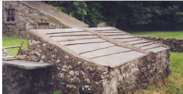
Fig. 38. In this example of single lap slating on a pigsty, the perpendicular joint is weathered with mortar. More commonly this gap is weathered by bedding a narrow slate over or underneath the joint. Photo: Terry Hughes.
