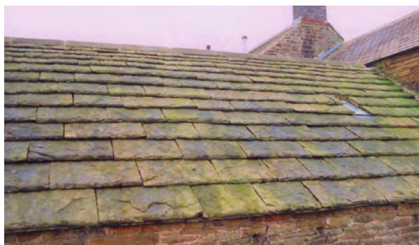
Fig. 21. Stone-slates from the majority of Carboniferous sandstone sources are flat and featureless. Some however, like this roof at Freebitch in Derbyshire, are more textured. At these delves it was common to dress off the rippled texture to allow them to lay well on the roof. Photo: Terry Hughes.
