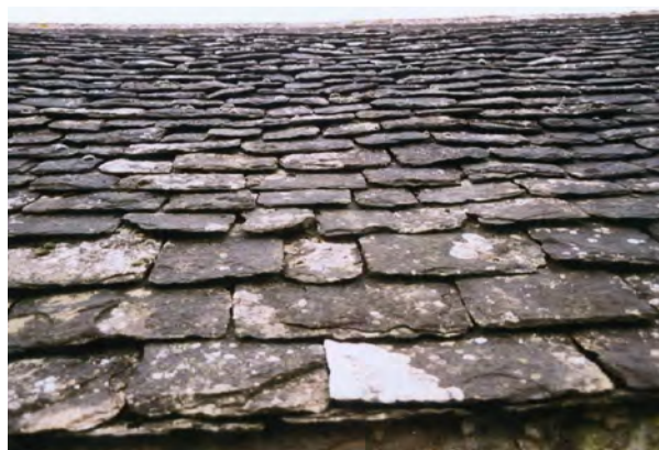
Fig. 29. At Stonesfield in Oxfordshire, Middle Jurassic pendle stone was frost split to produce thinner slates than presents such as those from the Forest Marble. The very thin frosted slates were desirable because of their lightness and have consequently been removed from local roofs for use on other buildings since at least the middle of the nineteenth century. Photo: Terry Hughes.
