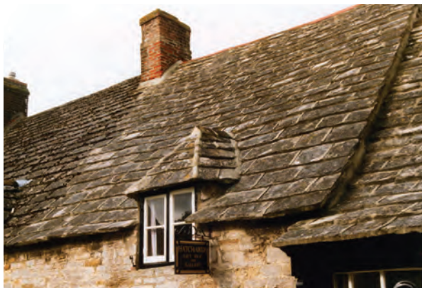
Fig. 32. In the Isle of Purbeck there is still a substantial stone-slate industry and generally the roofs are well conserved. Photo: Terry Hughes
