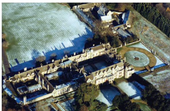
Fig. 31. The lack of new Collyweston slates has posed a serious problem for the conservation of buildings in the East Midlands and elsewhere for many years. It is hoped that the urgent need to substantially re-slate the roof of Apethorpe House will be the stimulus to re-establish production. Photo: English Heritage
