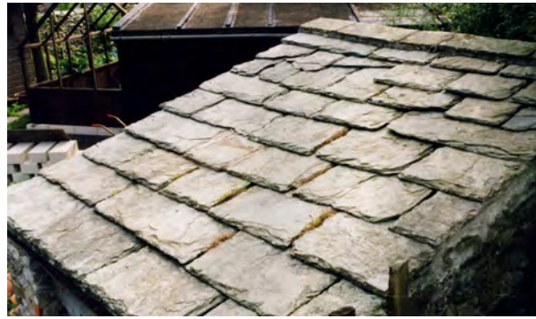
Fig. 9. The Ingleton slates from the Yorkshire Dales National Park had a purely local use. Long unavailable, the Park authority is trying to re-establish production. Photo: Terry Hughes
