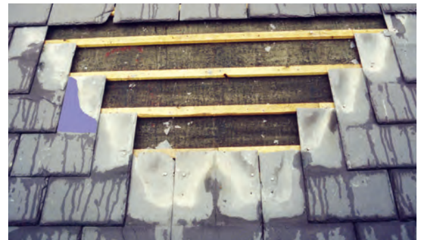
Fig. 34. Slate and stone roofs keep water out by having head and side laps large enough to prevent water passing over the top or round the sides of the slates. The area of water spread between the slates is an inverted T shape. In random sized slating, skill and experience is needed to select and position slates to achieve adequate laps. Photo: Terry Hughes
