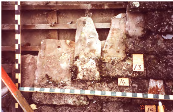
Fig. 17 Old Red Sandstone on the roof of Dore Abbey (Hertfordshire) during archaeological recording of the construction. A local initiative to obtain new stone-slates to repair the roof resulted in the establishment of three small delves. Photo: Terry Hughes
