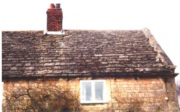
Fig. 24. A few Magnesian Limestone (Cadeby Formation) roofs have been identified in Nottinghamshire near Worksop. It is believed that in the past it was used over a much larger area. Today there are so few remaining roofs there is little prospect of re-establishing production. Photo: Terry Hughes
