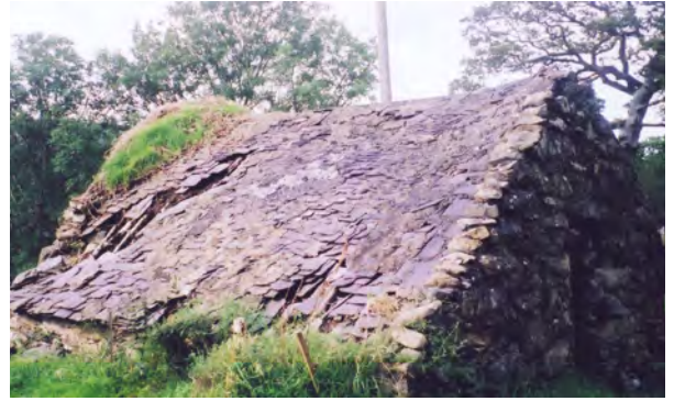
Fig. 5. The Welsh slate quarries have had a major influence on the roofscape of England. This example of Cambrian age 'pre-industrial' roofing slates pegged into turfs over oak wattling is from near Caernarfon in Gwynedd. Photo: Terry Hughes
