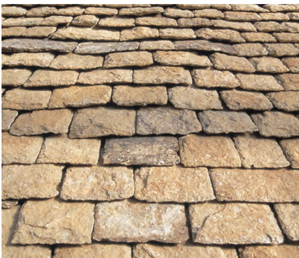
Fig. 12. The Harnage stone-slate roof of Pitchford Church in Shropshire. When slate or stone-slate production is being re-established, it is essential that a detailed specification for the product should be agreed with the delph operator. It should be based on a clear understanding of local tradition and cover criteria such as shape, size, shouldering, surface and edge dressing. Photo: English Heritage
