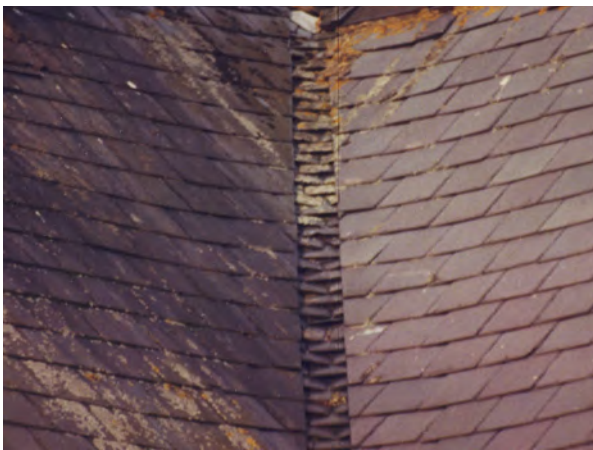
Fig. 50. Welsh valleys, which would once have been common in Wales and the Welsh Marches, are now rarely seen. This is a weak detail unless constructed with great care and skill and consequently is almost always replaced with an open lead valley. It is preferable to use the original detail but with the inclusion of a lead soaker in every course. Photo: Terry Hughes.
