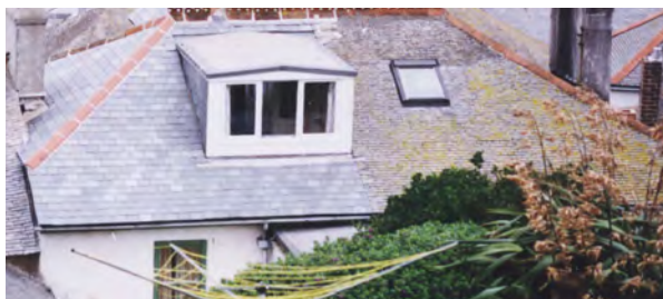
Fig. 18. Traditional, Old Delabole slates like those on the right side of this roof are often replaced by slates of a different format and/or from other sources. In this example, small, random, Cornish slates have been replaced with large, single sized, Brazilian. Where conservation is important, it is essential to ensure the correct format is selected (small, random, etc) as well as the traditional source. Photo: English Heritage
