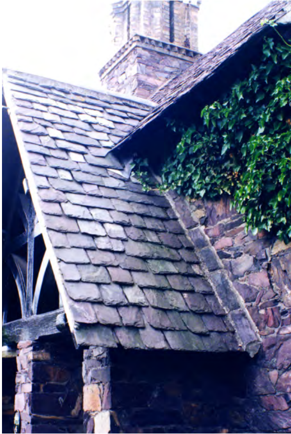
Fig. 4. The Swithland slates of Leicestershire produce distinctive roofs which cannot be accurately conserved because production ceased in the early nineteenth century. Photo: Terry Hughes
