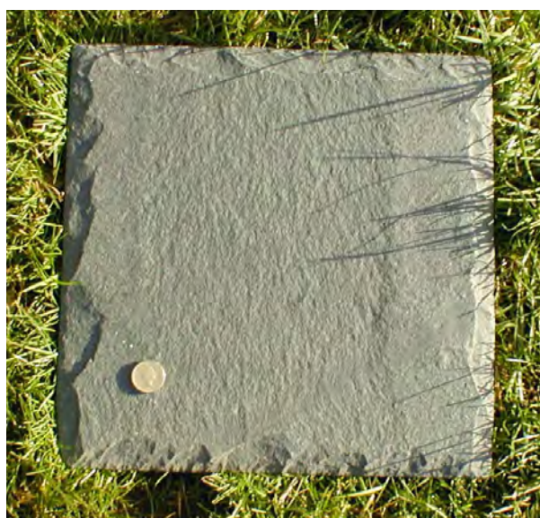
Fig. 15. The Burlington Blue Grey slates are an important roofing material regionally and nationally. Provided care is taken with the specification, there is no difficulty in conserving these roofs. Photo: Terry Hughes
