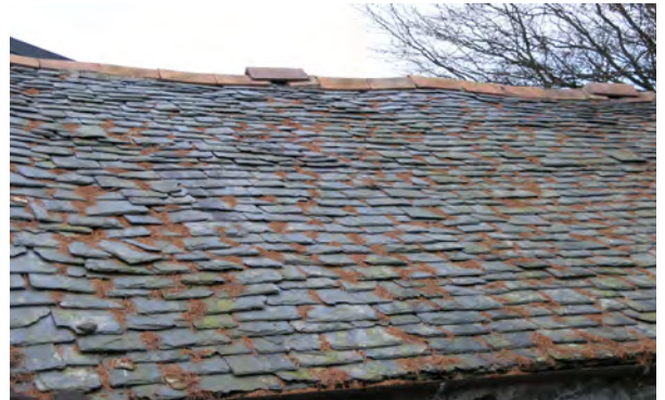
Fig. 6. Ordovician age slates near Corwen in North Wales. Vernacular slates and stone-slates are random sized and are arranged on the roof with diminishing lengths up the roof slope. Photo: Clwyd County Borough Council.
