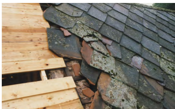
Fig. 23. In Dumfriesshire, the Permian age red sandstone, similar to that of the Eden Valley in Cumbria, has been used for an ancient roofing style: diamond pattern slating. This was the way Roman stone or slate roofs were constructed. Photo: Terry Hughes
