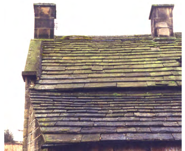
Fig. 20. A Carboniferous age sandstone roof in Derbyshire. The Millstone Grit and Coal Measures groups produced roofing throughout the uplands of northern England. In the Lancashire – Yorkshire industrial belt, together with production of flagstones for flooring, this developed into a major industry in the nineteenth century. Photo: Terry Hughes
