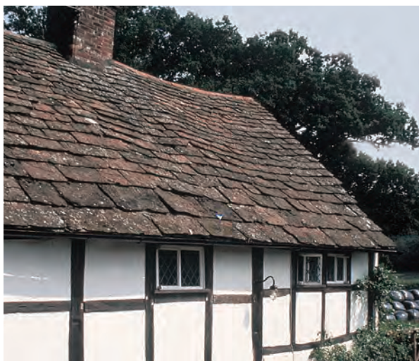
Fig. 33. The conservation of Horsham stone roofs has been under great difficulty since production ceased in the 1930s. Happily a new delph has recently been opened and shows signs of being commercially successful. Photo: English Heritage
