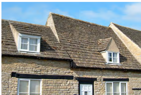
Fig. 30. A typical limestone roof near Stamford in Lincolnshire. The small sizes of these random sized Collyweston slates can be easily laid to raking intersections and curves making it easier to construct hips, valleys and small dormer roofs. Photo: Terry Hughes
