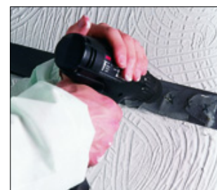
Drill through paste. Duct tape will prevent the edges from crumbling
