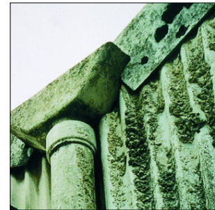
Moss and lichen growth on asbestos cement
